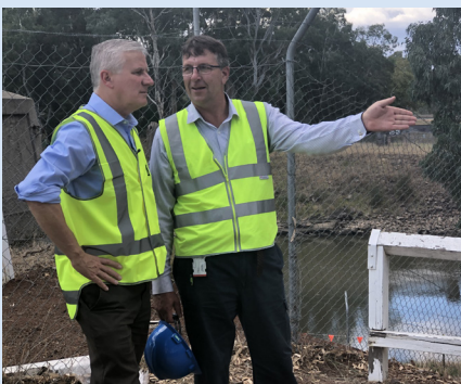
PROTECTING WAGGA WAGGA: Inspecting levee bank upgrade work in March with Wagga Wagga City Council Senior Project Manager Darryl Woods.
