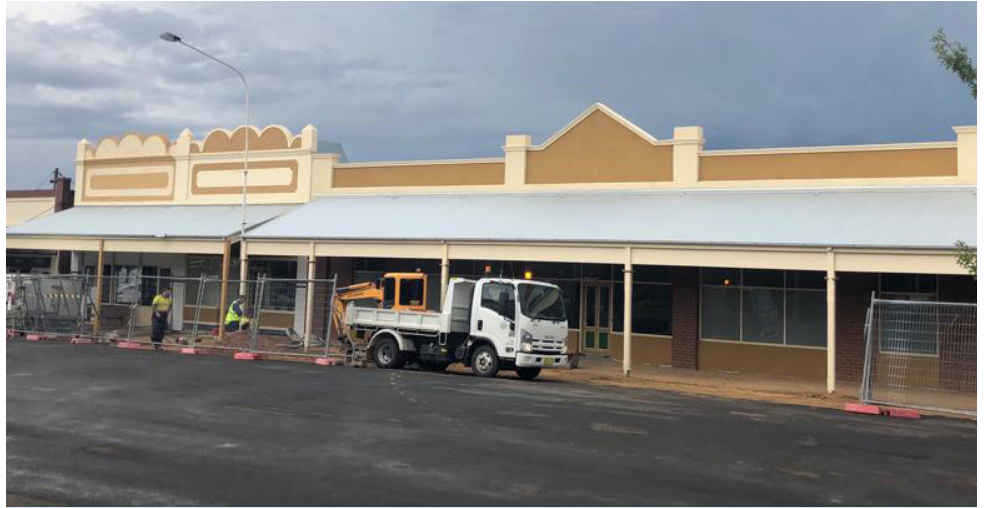
BUILDING BETTER HEALTH: The new Grenfell medical centre under construction.
